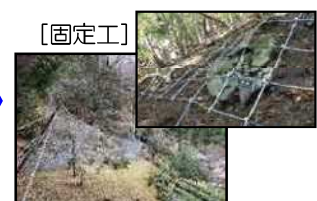
[固定工] [落石防護柵工]
