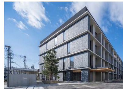
Construction of prefectural facilities
