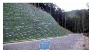
Paving of forest roads
