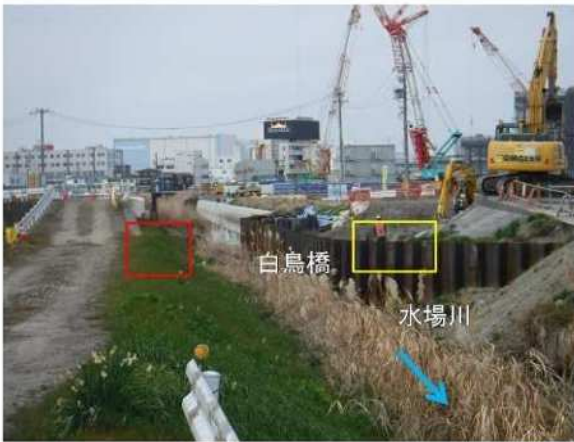
③水場川：橋梁改築、河道整備、調節池整備
